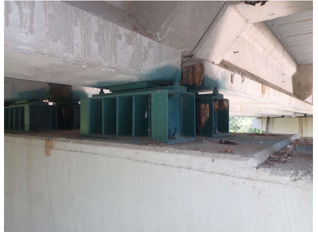
Bent 3 Bearings on Pedestals
