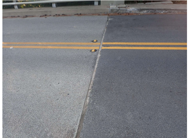
Joint intact, copolymer overlay intact
