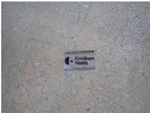
Crack in Curb
