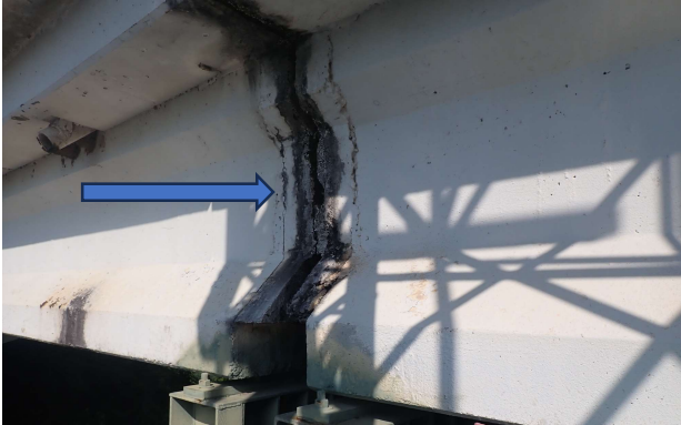
Cracking at Edge Beam
