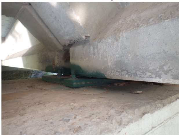
Bent 2 Bearings
