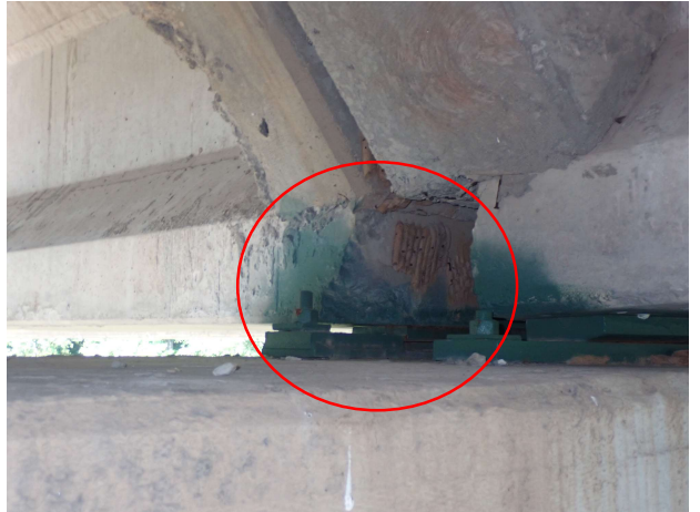
Beam 2 Span 3 corner spall
