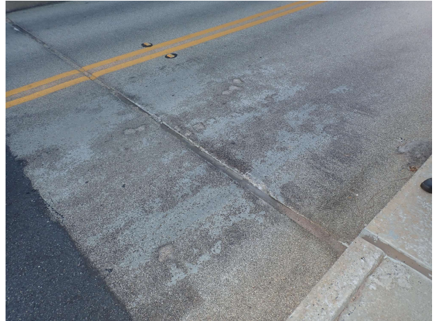
Overlay Damage
