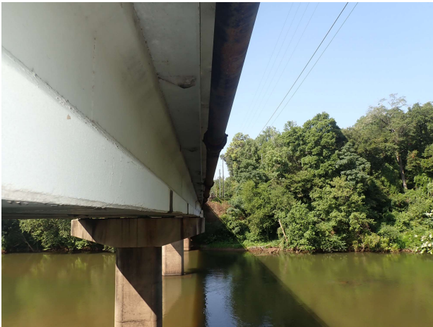
Utility, sewer on left overhang
