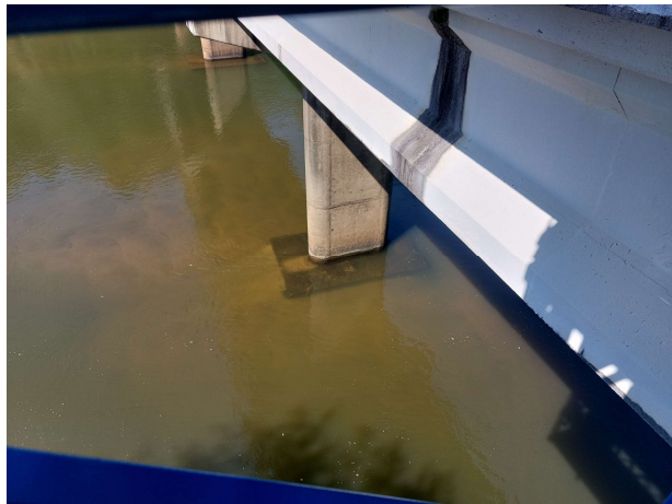
Silt around footing covers seal
